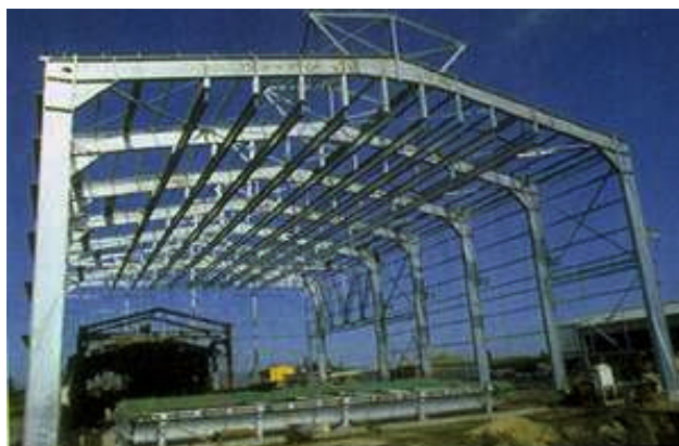
Galvanised steel building framework
